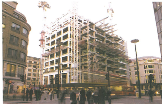
Steel beams make taller structures possible.
